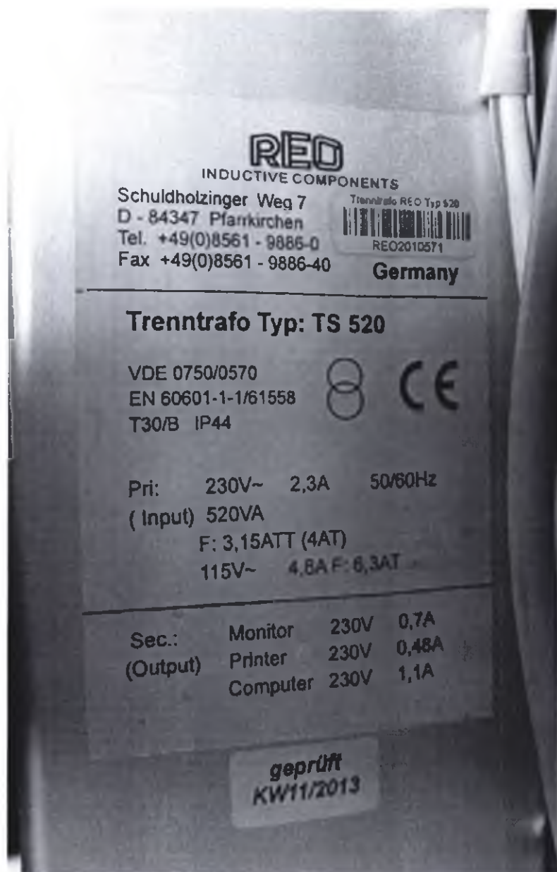
Image 7. Main marking label on the Isolating Transformer.
