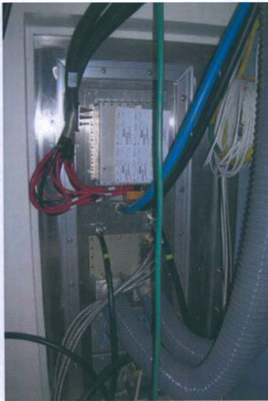
Utility Room Side
