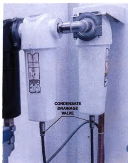
Figure 12.1 – Filters, installed in SEC 7HC adsorption dryer (from left to right: cyclone, micron, submicron)
