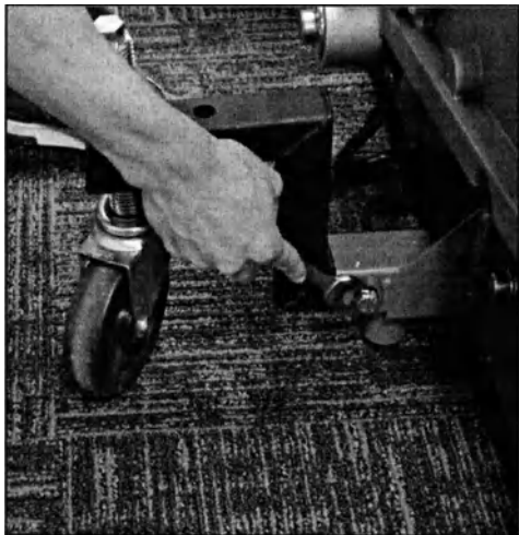
Figure 3 – Unscrew Tube \frac{1}{4} Screw (6.35 mm)
